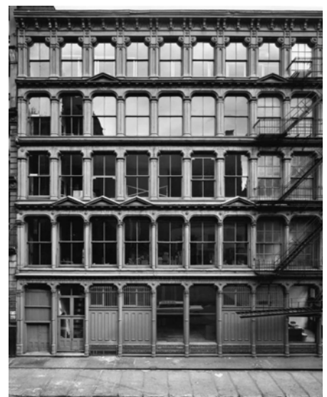
Donald Judd's studios at 101 Spring Street in New York - a cast-iron building designed by Nicholas Whyte in 1870. Judd wrote in 1989 that the facade of the building "is the most shallow perhaps of any in the area and so is the furthest forerunner of the curtain wall".
