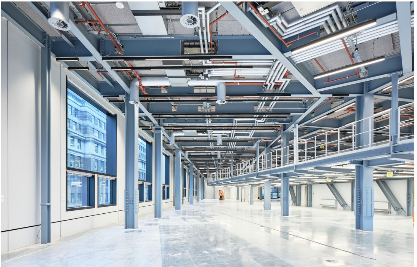
Retained floor with mezzanine and acoustic panels mounted above services
