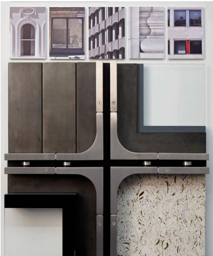
Sample board with the machined junction of the cladding frame
