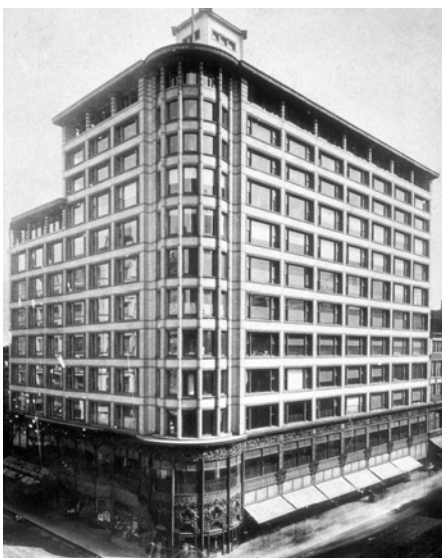
The Carson Pirie Scott & Co. department store, Chicago, 1899, designed by Louis Sullivan and Daniel Burnham, has deep reveals across the facade that give a sense of solidity despite the large windows.
